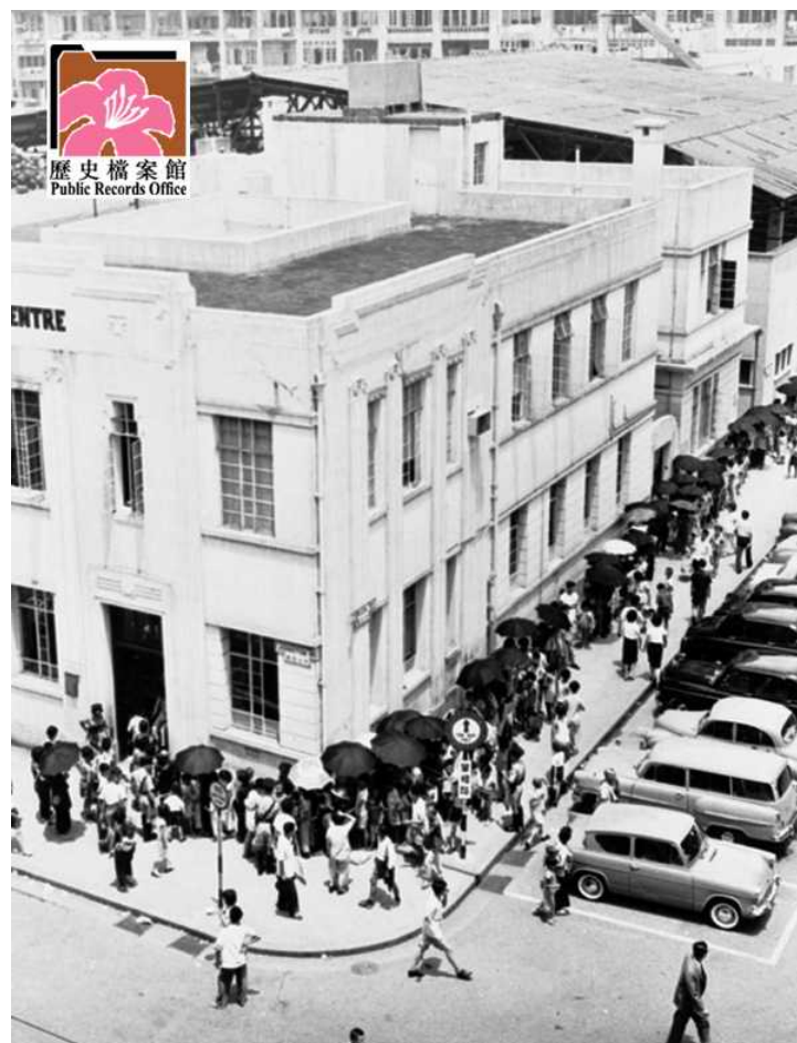
Figure 2: Violet Peel Health Centre in 1961. Opened in 1935 and designed by Chau & Lee Architects. (Item HKRS365-1-78-4, Public Records Office, Hong Kong)
