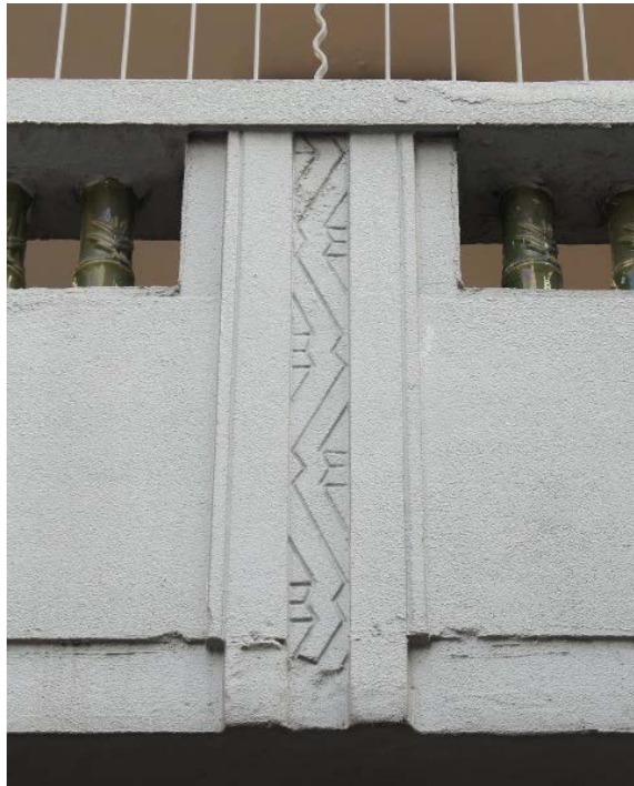
Figure 4: Stylized sunbursts and zigzag moulding flanked by bamboo-grilles at the balustrade of the Dispensary (Photograph by author)
